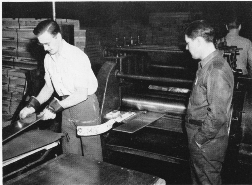
Joe Lokis is handling one end of a flat brass metal that has just come through a straightening roll in the North Mill. Charles M. Pranulis, maintenance man, looks on. Charlie suggested the idea of bending and twisting a flat steel bar (painted white) to form a guard and brace for the man on the receiving end of the rolls.
